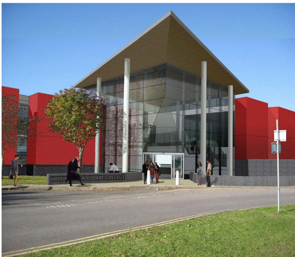
A view of the proposed new entrance to the Flackwell Heath campus
